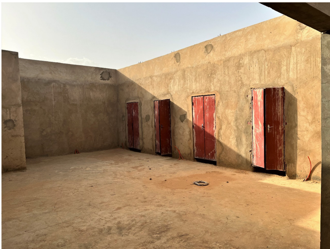
Picture 3 – Unfinished craft workshop building at the end of the contract
